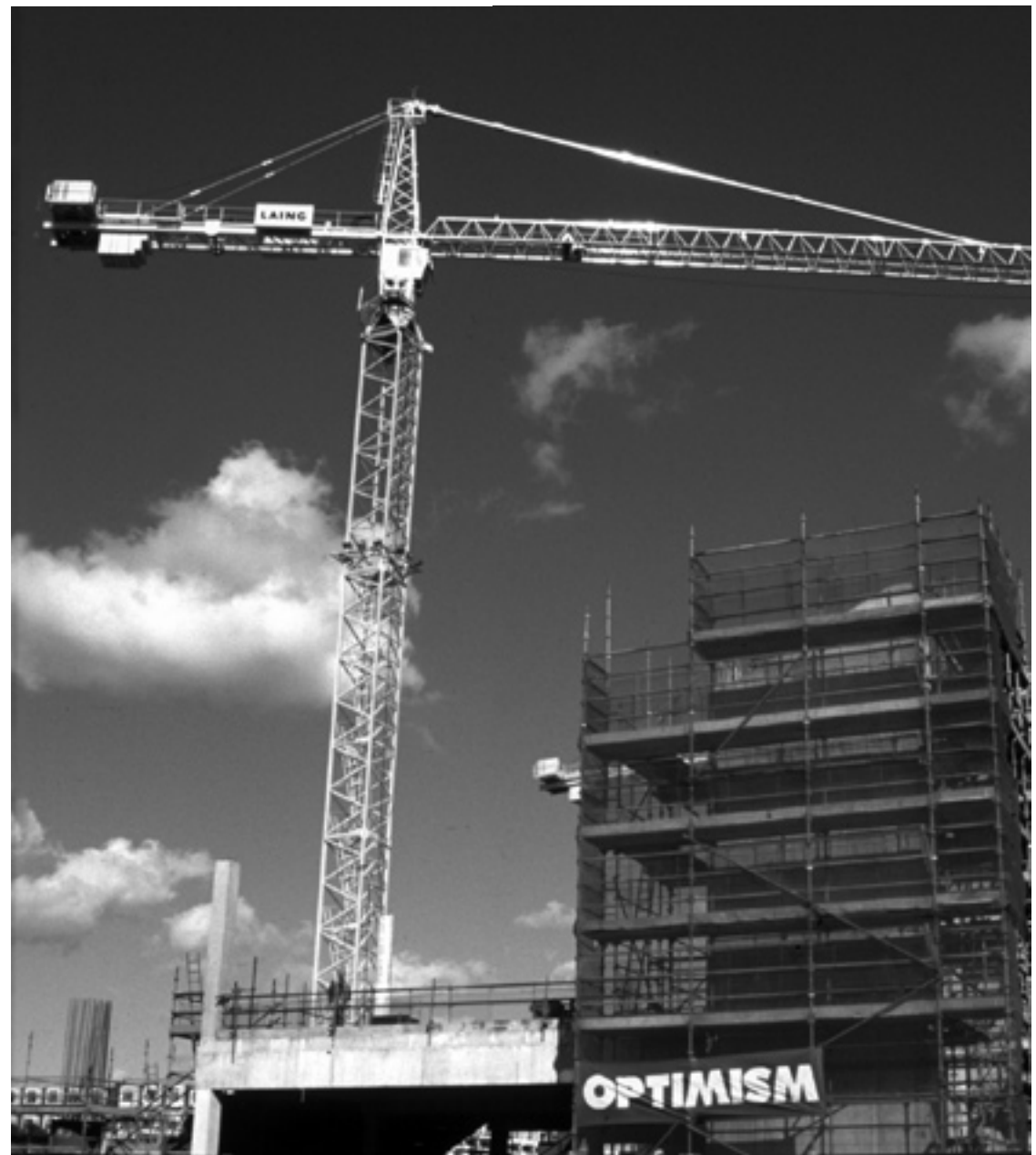
Ryan Gander, Banner for Europe, 1999. A banner on the building site for the commonwealth games swimming pool, Oxford Road, Manchester, UK.
